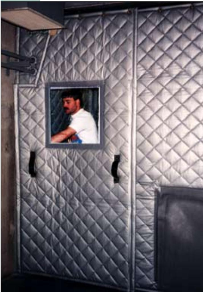
The door panel allows easy access to the chiller. A "drop-down" view window provides immediate access to control knobs.
