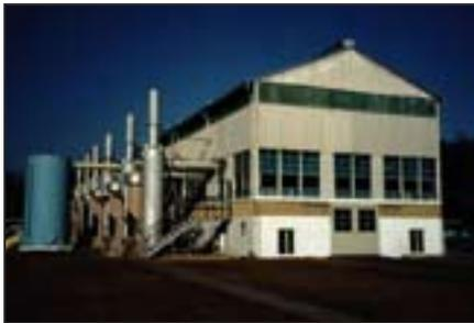
Tennessee Gas Pipeline's mainline compressor station houses five 1400 horsepower compressors.
