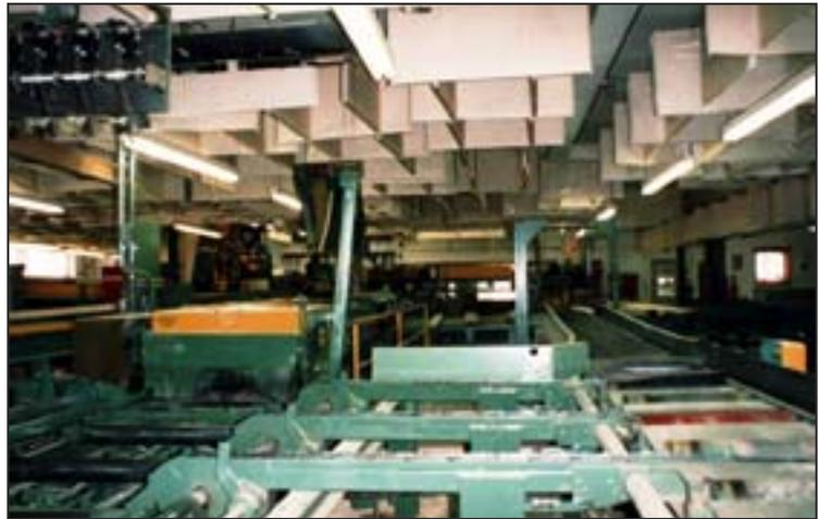
High NRC, low-cost, Class A flammability rated Sound Seal polywrap baffles installed throughout the wood working facility.
